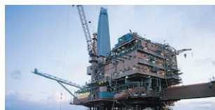
Oil and gas (up-, mid- and downstream)
