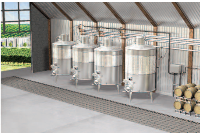
Winery fermentation tanks with thermal jackets
