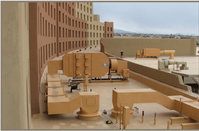
Sandia Resort & Casino installation
