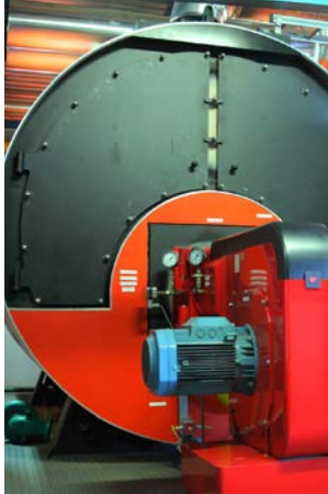
Combustion-Burner/Boiler
